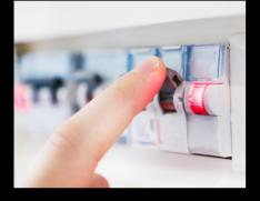
From the meter, cables run out to your consumer unit (often referred to as a fuse box).This contains the main on/off switch and a number of miniature circuit breakers (MCBs), which protect individual circuits. An MCB will automatically disconnect the supply of electricity if one of the circuits is overloaded or if there is a fault. You can reset an MCB by simply switching it back to the 'on' position.
